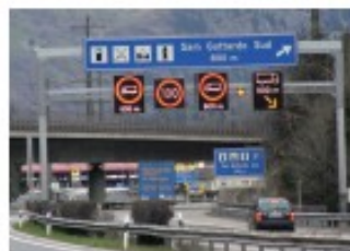
→ ...as installed at the Gotthard Tunnel
